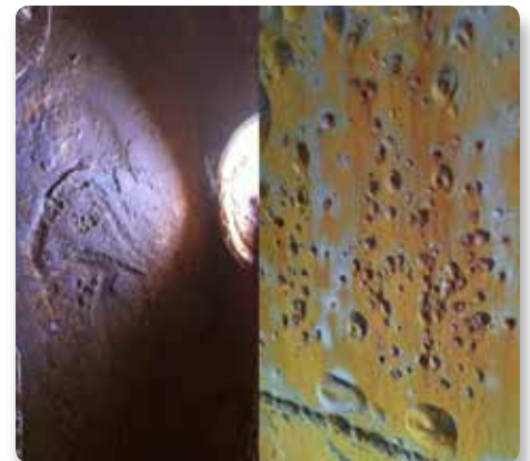
No Surface prep, Tank Lining Corrosion caused by bacteria
